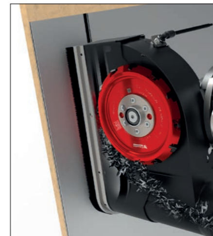
V-GROOVING ON ACM
